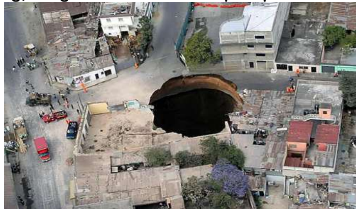
[Guatemala, also Florida sinkholes]
